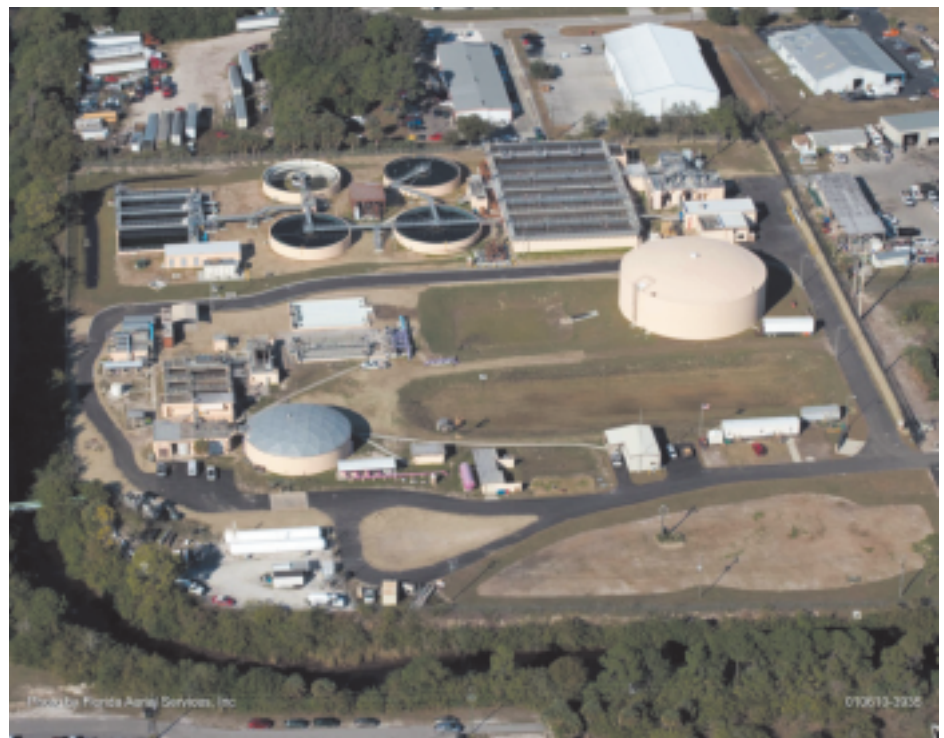
Figure 3. Upgraded Wastewater Treatment Facility (Florida Aerial Services Inc., January 2010)
